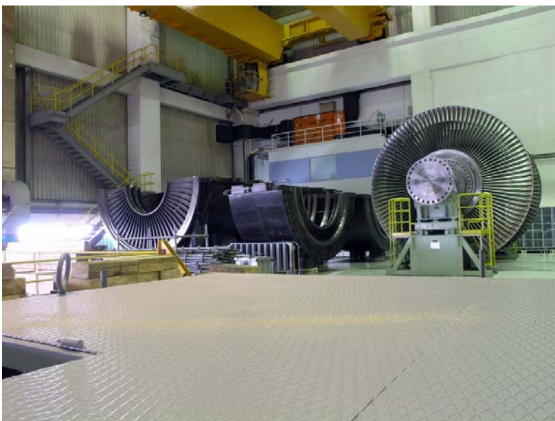
Figure 16: Replacement of low pressure turbines during the refueling outage 2006.
